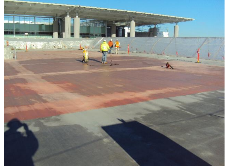
RCF Level 5 Traffic Coating Application
