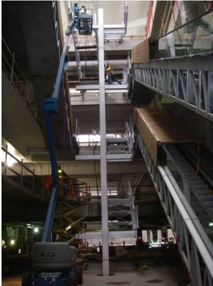
CSB Architectural Stair K Progress
