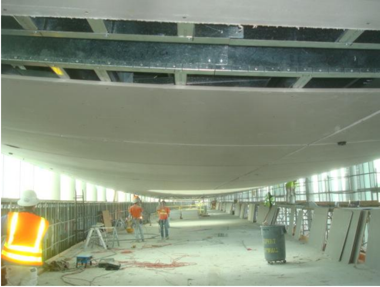
CSB Vaulted Ceiling Installation Progress
