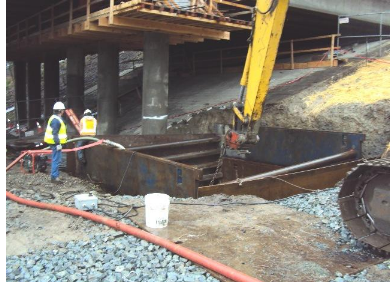
ORI SR99 Bridge Widening Pier 2
